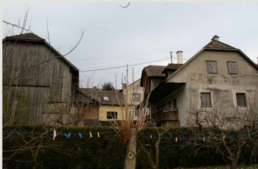
Garden view prior to renovation
